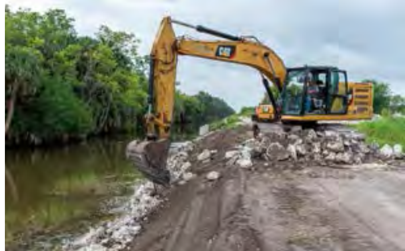
Regrading the levee slopes along the Lake Apopka Wildlife Drive (top). Stabilizing the levee on the Apopka-Beauclair Canal (bottom).
