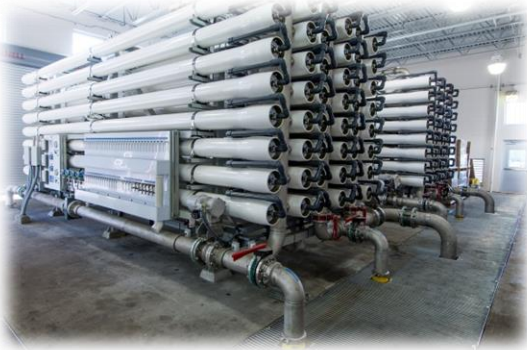
Reverse osmosis membrane unit in Palm Coast, left. Water storage tank in St. Johns County, right.
