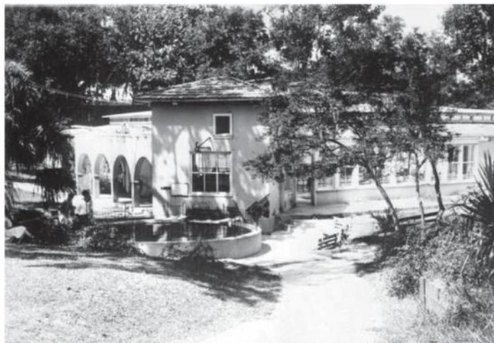
Figure 5. Green Cove Spring, the enclosed circular feature in the left middle, and casino in 1929. Photograph by Herman Gunter courtesy of the Florida State Library and Archives.
