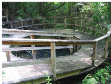
Figure 22. Structure surrounding W. W. Gay Spring #1.
