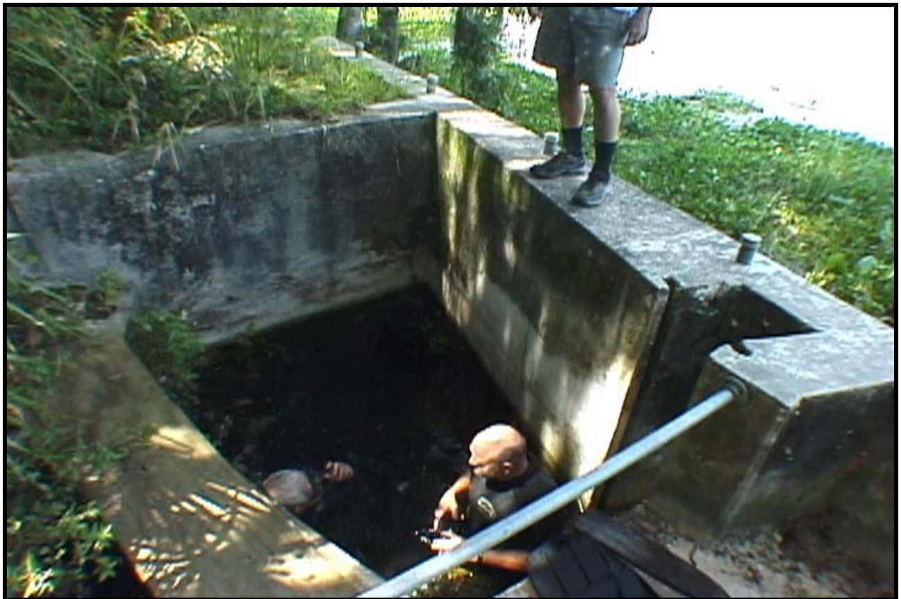
Figure 7. Video still of Sim's Spring, Marion County, Florida. The apparent vent is under the concrete wall on the left. The vertical slot behind the diver on the right is a discharge control structure.
