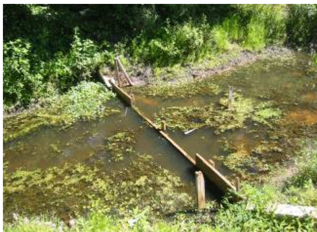
April 2005. Damaged weir
