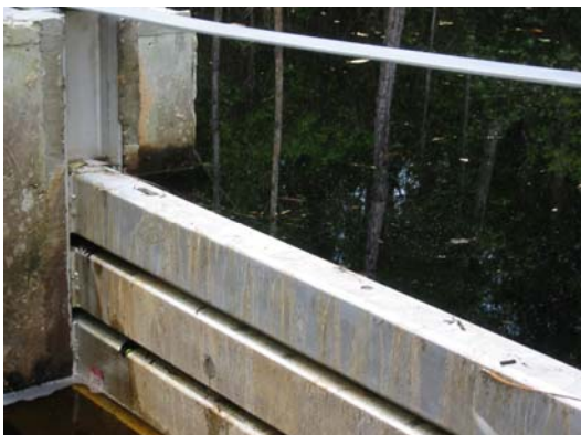
Control weir elevation 26.4 NAVD88 (27.5 feet NGVD29)
