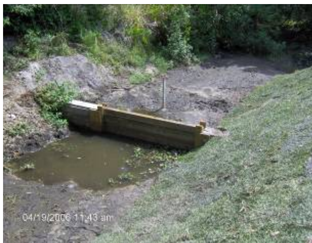
April 2006. Repaired and reinforced weir
