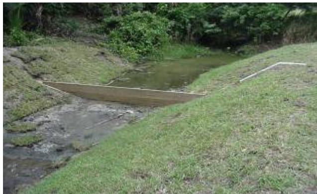
April 2002. Newly constructed outlet control weir in the Parkland Street ditch
