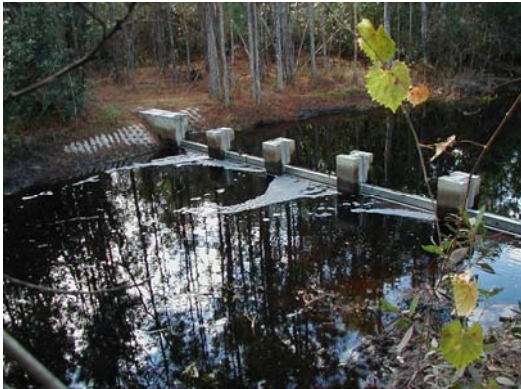
Weir with newly installed stop-log boards, February 2004.
