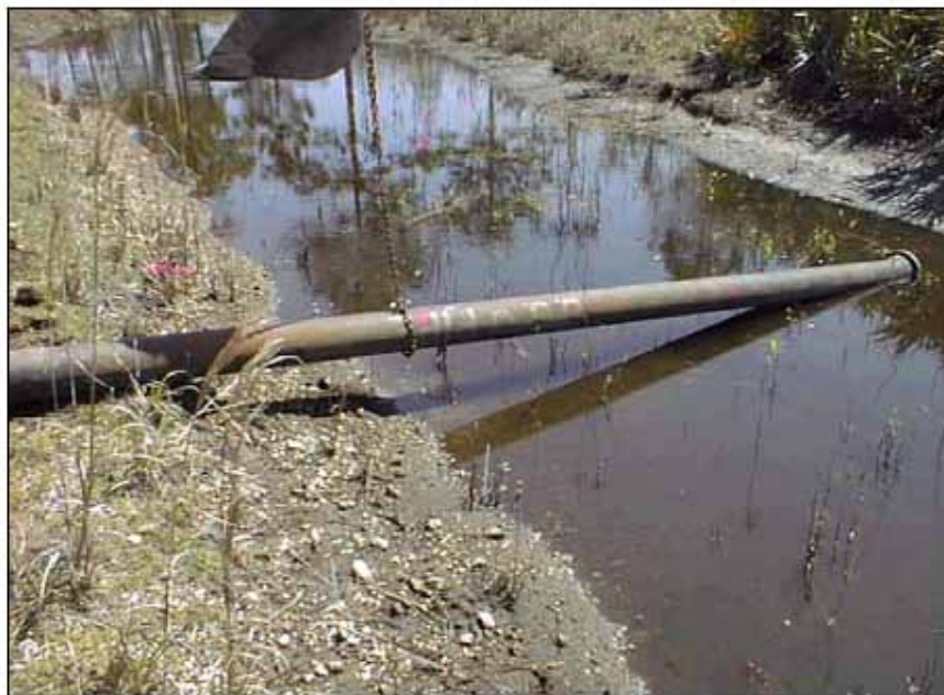
Figure 4. Construction of groundwater delivery pipe to Port Orange Wetland
