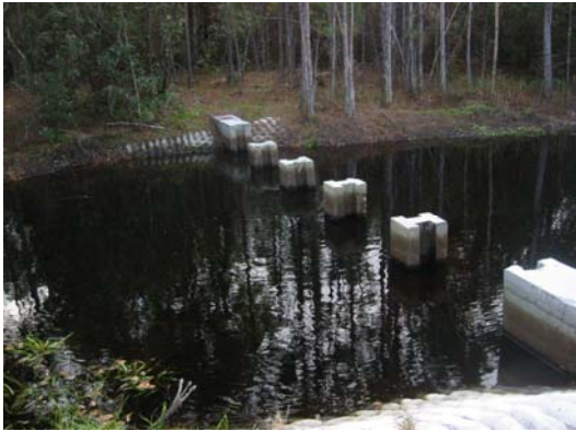
Weir under construction, December 2003.
