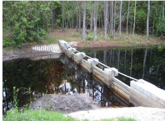
Another board added to bring weir to correct height, April 2004.
