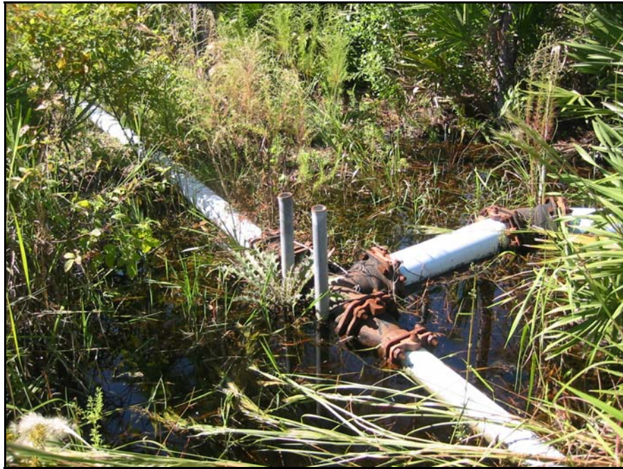
Figure 5. Diffuser pipe (left foreground) and “T” from delivery pipe (right-center)
