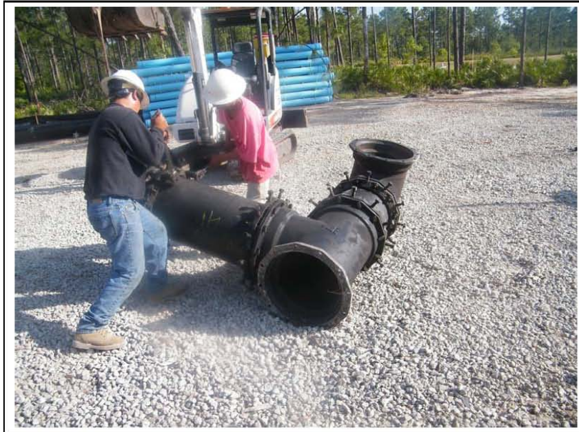
16" Pipe and Fittings Assembly
