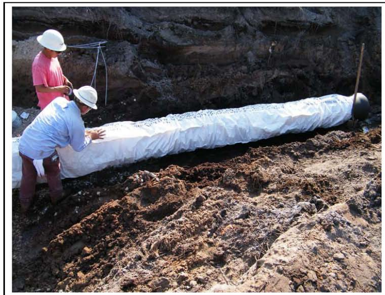
16" DIP Water Main Installation
