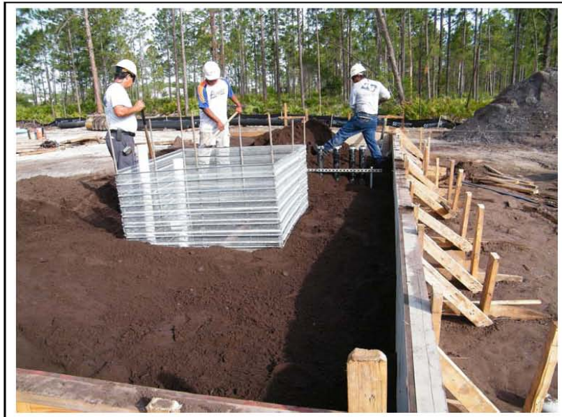
Concrete Pad Foundation and Form Work
