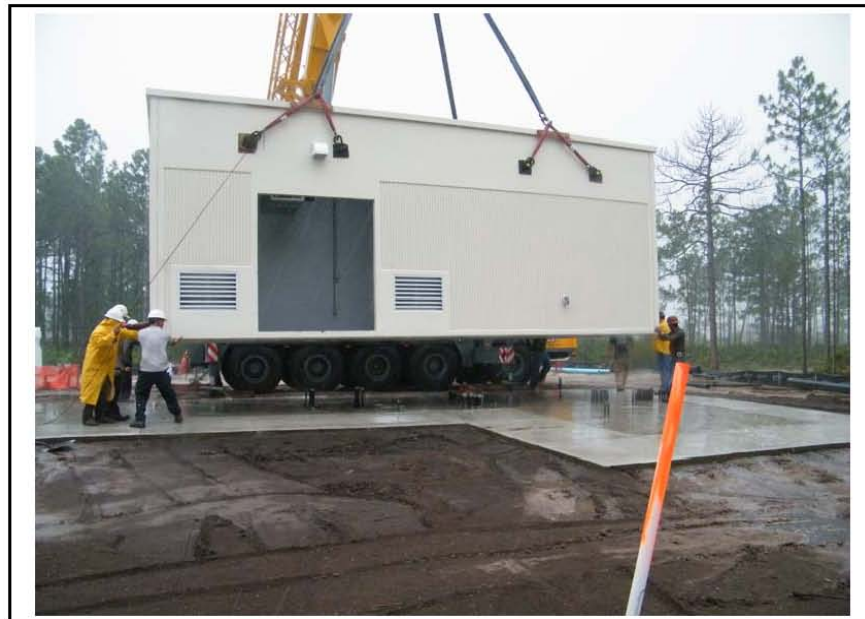
Pre-Fabricated Concrete Building Placement
