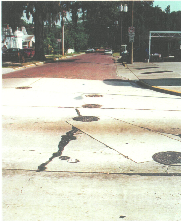
Mills Avenue and Minnesota Street intersection. Drainage well is located beneath street.
