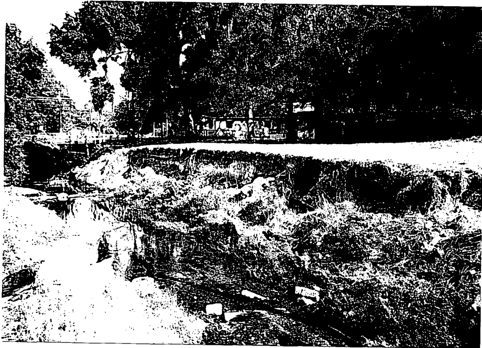
(Downstream of Kelvington Drive bridge, Orange County)
