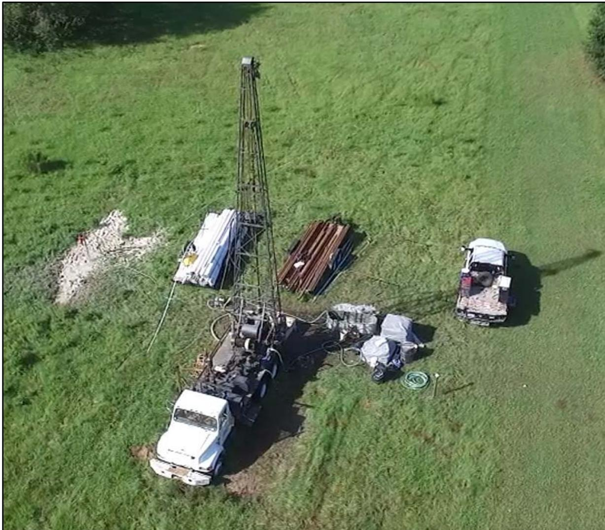
Figure 14. UAV view of drill rig and equipment used to construct monitor wells for water level monitoring and dye sampling.
