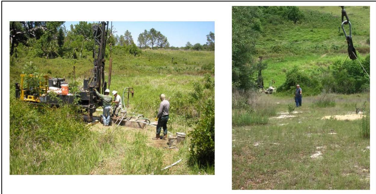
Figure 5. Track mounted drilling rig used to drill the test hole in the bottom of the sinkhole (left image). Right image shows District staff John Lombardi deploying the cable from the geophysical logging truck stationed at the rim of the sink.
